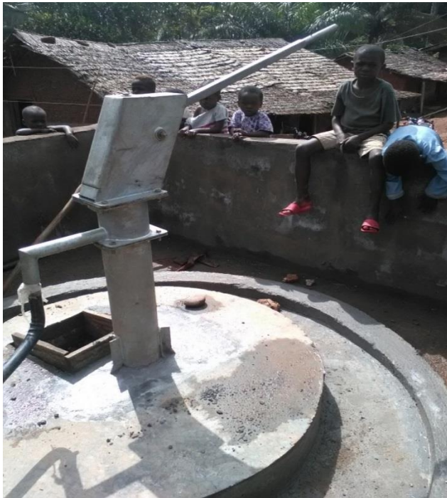
Borehole and hand pump under construction
