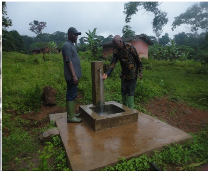
Tap functioning well but surrounding dirty
